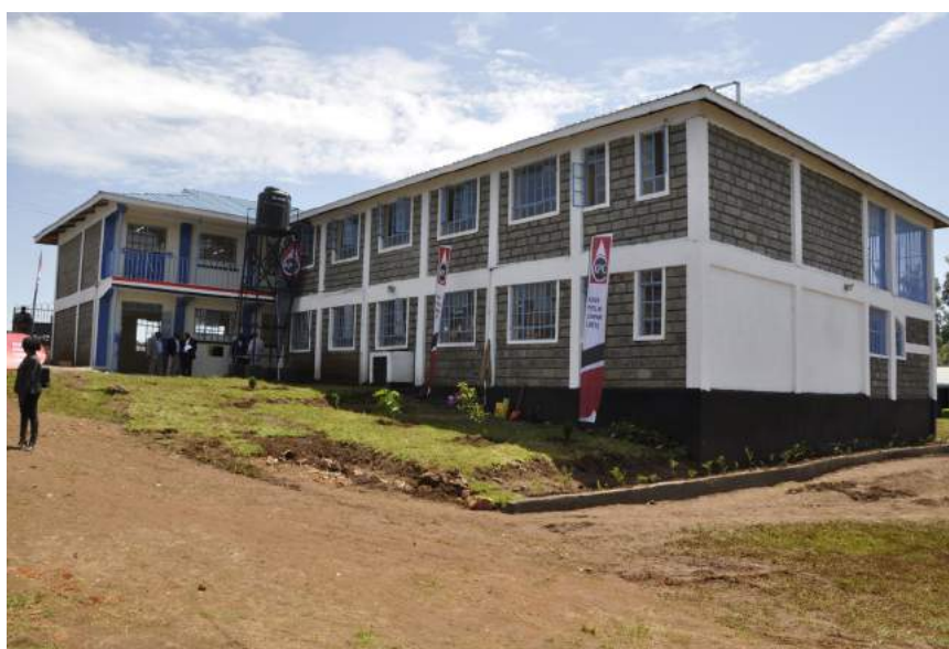
Construction of 4No.classrooms 1 storey block at Cheptuiyet Girls High School was done by KPC Foundation.
