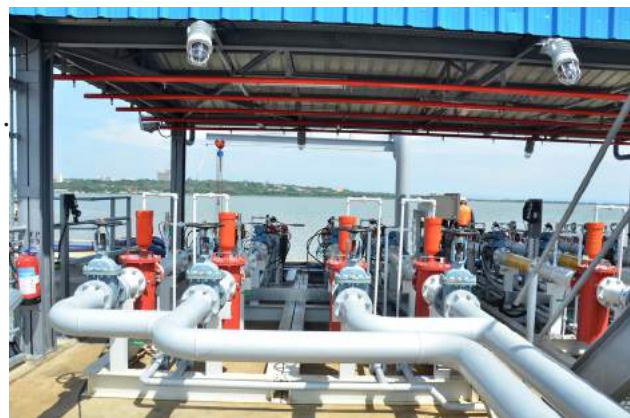
The completed Kisumu Oil Jetty.
