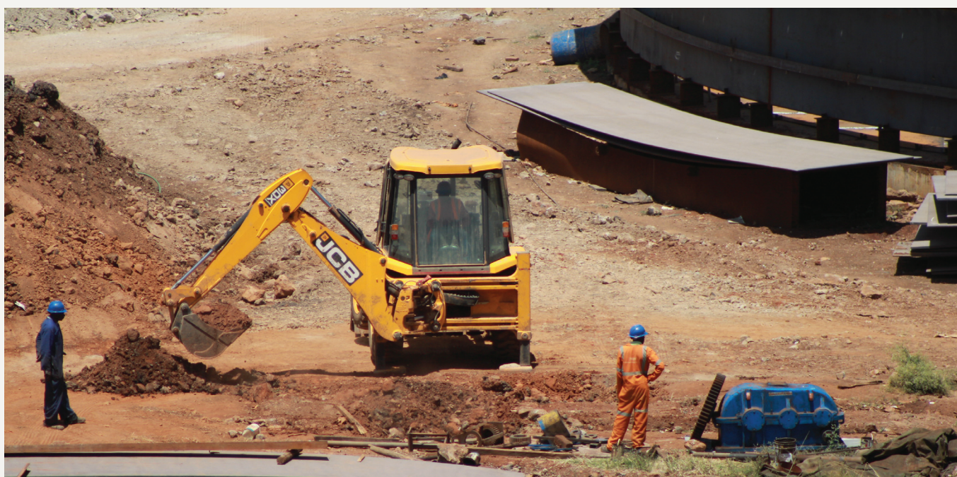
» Constructions works of additional storage tanks at Nairobi terminal.
